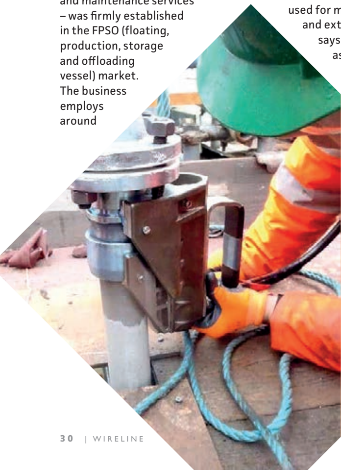
Lokring flanges installed on site
